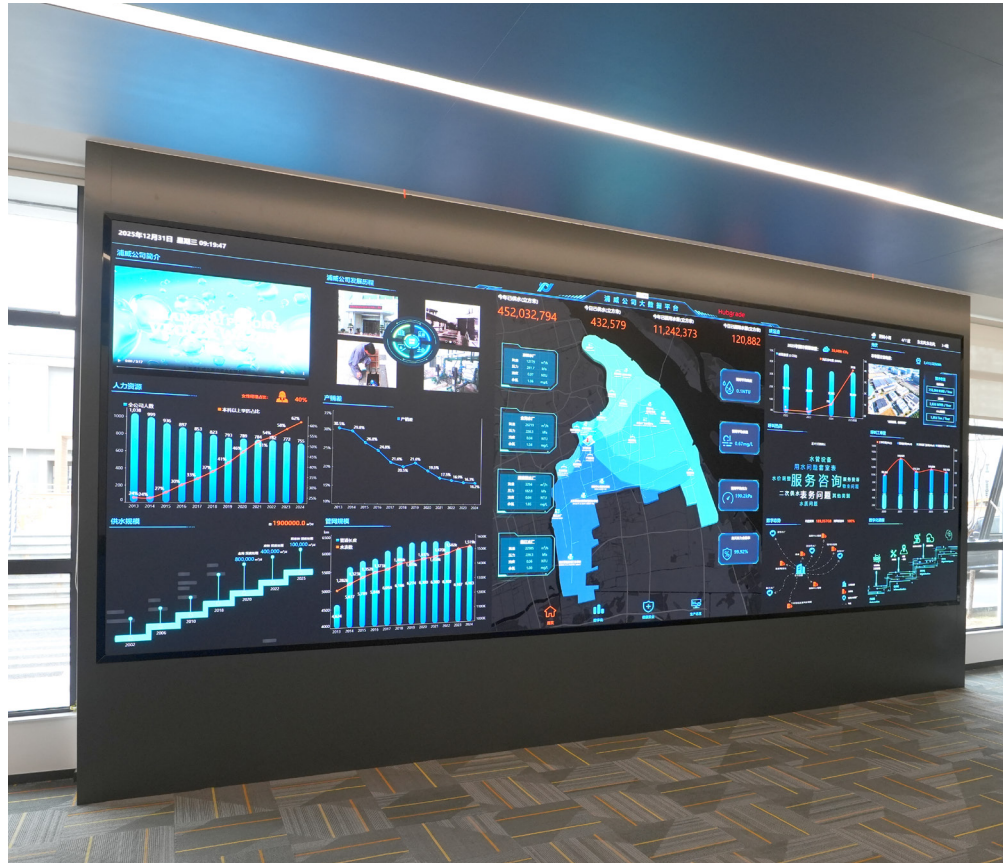
Shanghai Pudong Municipal Water Plant Project
