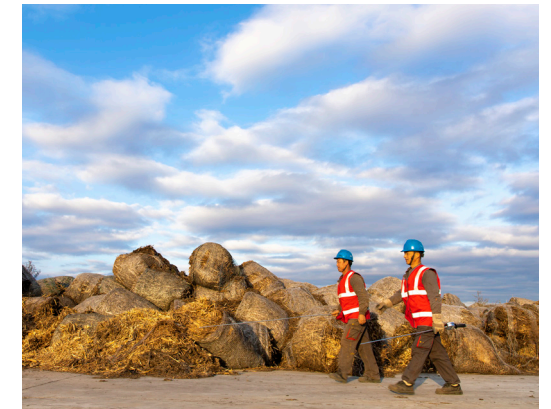
📍 Heilongjia Kedong Biomass Heating Project
