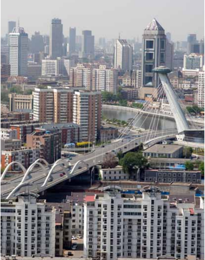
Veolia works closely with the Tianjin municipality to supply three million of the city's inhabitants with drinking water and to treat hazardous waste.
